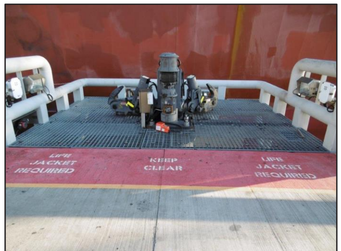
Figure 3: Mooring Hooks on Outer Wharf
